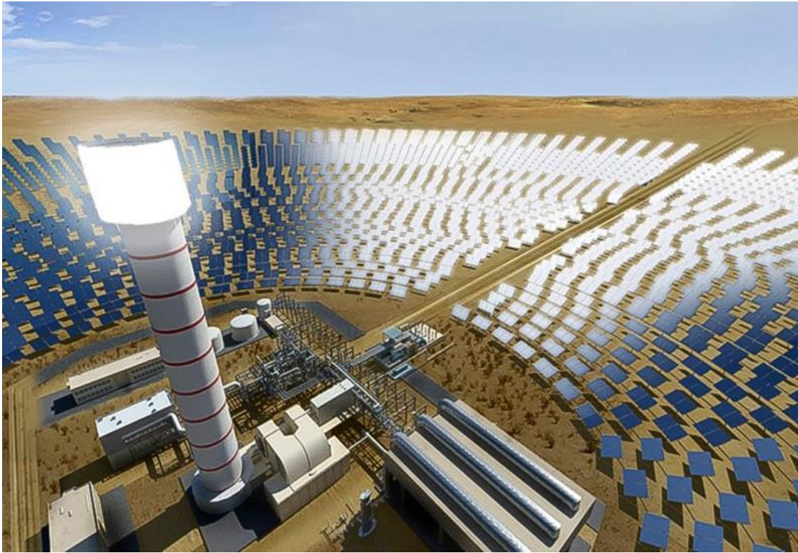
World's largest CSP in Dubai
